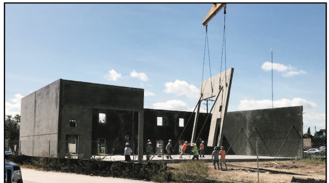
A solid concrete tilt-up wall is placed in position.
